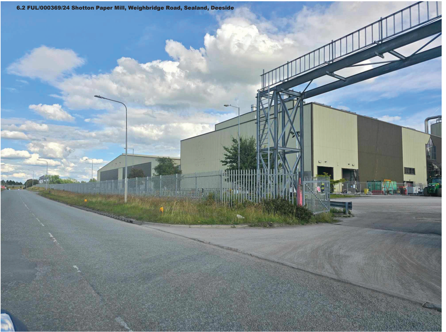
6.2 FUL/000369/24 Shotton Paper Mill, Weighbridge Road, Sealand, Deeside
